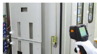
Temperature inspection of a clean room distribution board
