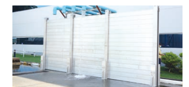
Flood wall assembly training at the manufacturing site in Thailand
