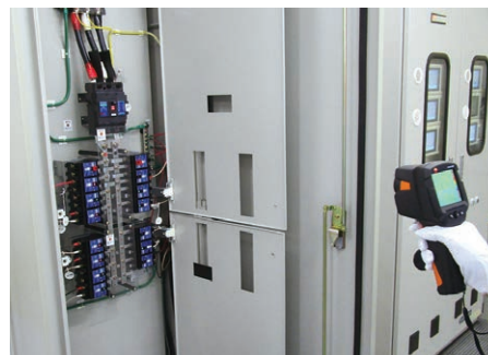
Temperature inspection of a clean room distri- bution board
